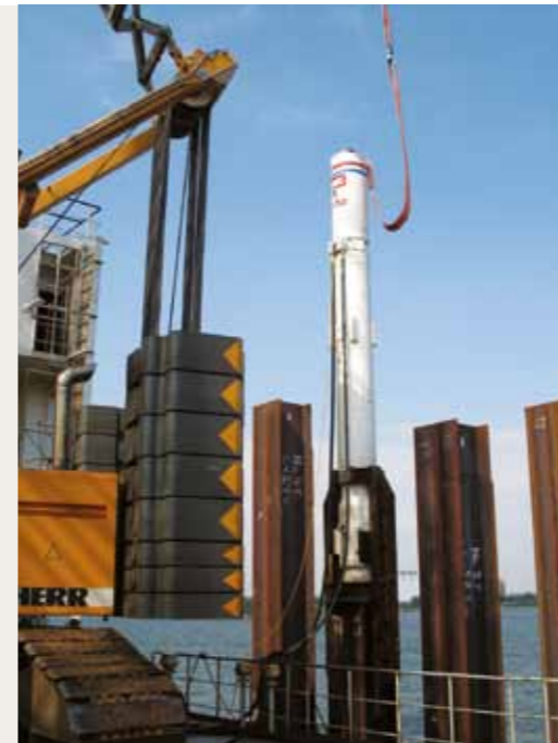
Coverage with the polygonal anvil at the profile L25
