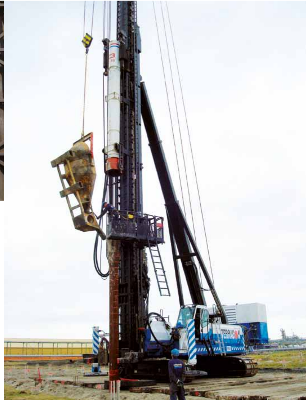
Driving Cast-In-Situ piles
